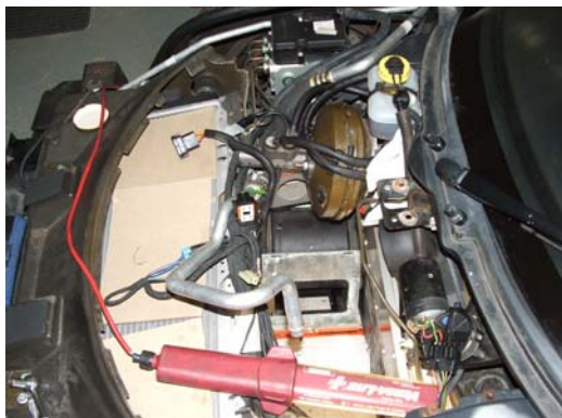
Blower unit is located under the chassis rail
