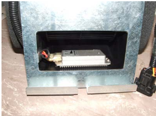
Speed control unit mounted inside blower
