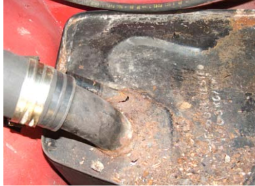
Corrosion caused by water soaked foam
